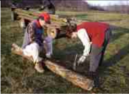
Doug and Catherine work on a bridge
