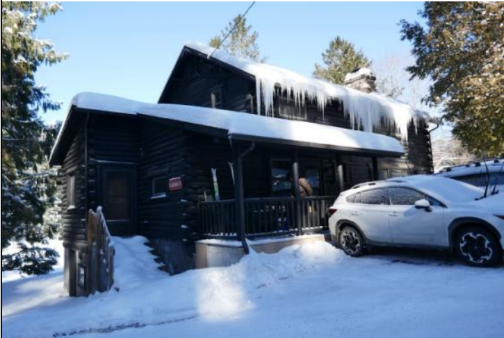
Cabin 11, the former HQ of the CCC built in 1936 photo by Marcie Schubert
